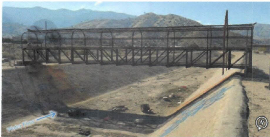
Figure 2-36. School Pedestrian Bridge (Non-Project), Looking Downstream (Photo Date: 01/2020)
